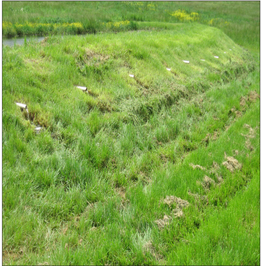
Figure 3. Slow release of water from weep berm outlet to grassed riparian zone.
