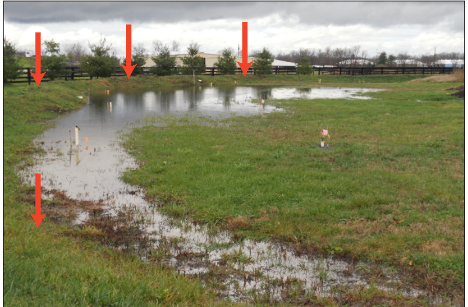
Figure 2. Red arrows point to a contour weep berm installed on a horse farm.
