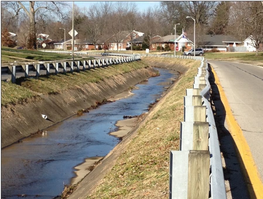
Figure 5. Conventional stormwater management is designed to collect and rapidly convey runoff to streams, some of which have been lined with concrete because they eroded so badly.
