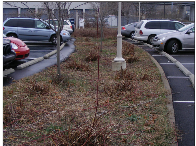
Figure 11. Parking medians, such as this one at the Sanitation District 1 parking lot in Northern Kentucky, are ideal locations for bioswales. Photo courtesy of Jim Hansen of EcoGro.
