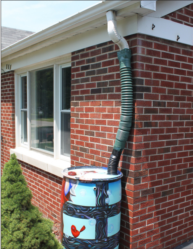
Figure 7. Rain barrels are ideal for collecting rain water from roof tops for future use.
