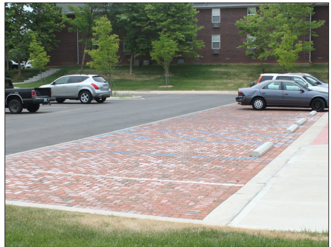
Figure 10. Permeable pavement, such as these interlocking clay brick pavers, is ideal for light traffic areas such as parking lots.
