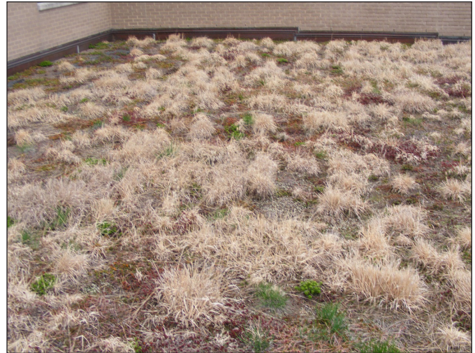
Figure 9. Green roofs, such as this one, help reduce runoff volume and reduce the building's energy usage.
