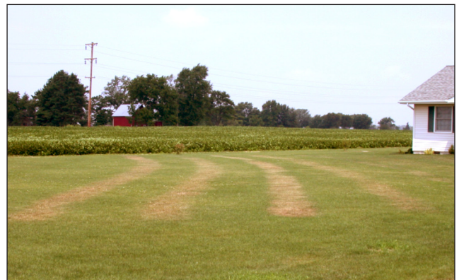
Figure 1. Brown turfgrass over soil absorption field trenches indicates an absorption field that is probably functioning as designed.
