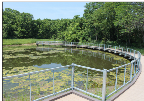
Figure 1. Stormwater wetlands, such as this one at McConnell Springs in Lexington, Ky., help improve stormwater quality while providing an educational opportunity for citizens.
