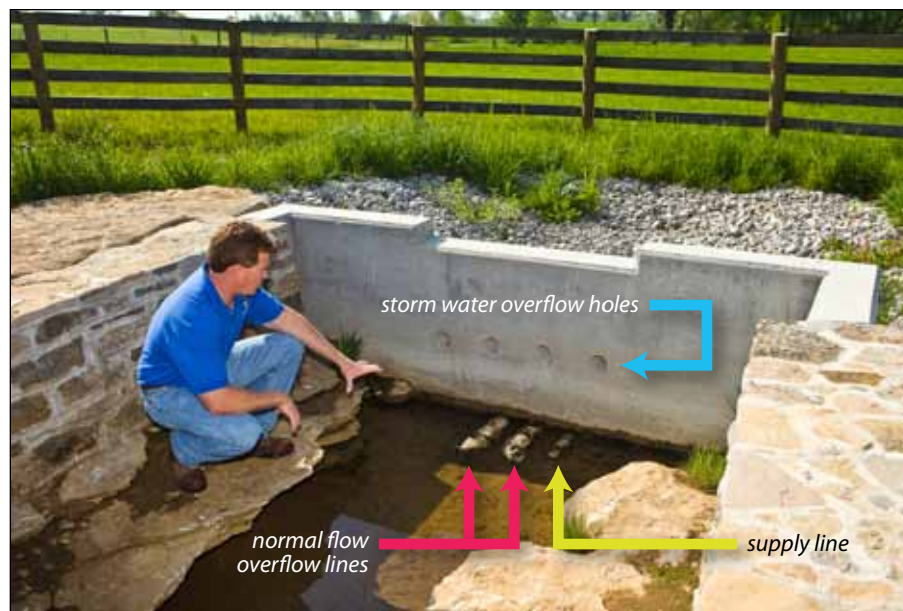
Figure 1. This developed spring provides an alternative water source for livestock.
