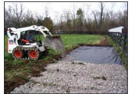
Figure 5. Base layer of crushed stone.
