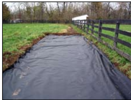
Figure 3. Geotextile fabric in place after excavation.
