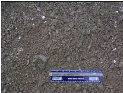
Figure 8. Densely graded aggregate for the surface layer.
