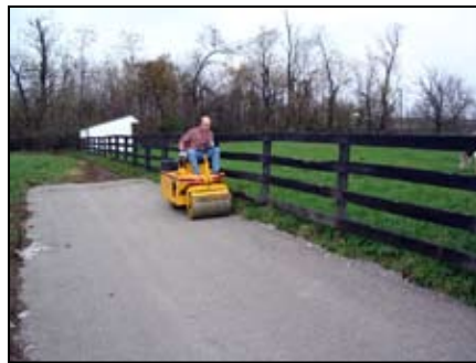
Figure 9. Compaction with drum roller.
